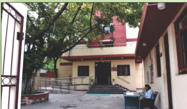
Hostel Main Entry Gate
