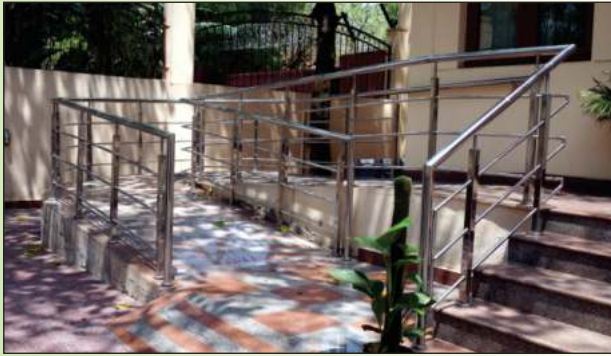
Ramp for PWD Residents
