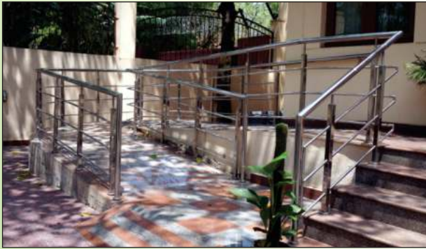
Ramp for PWD Residents
