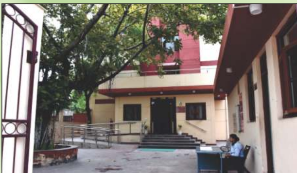
Hostel Main Entry Gate
